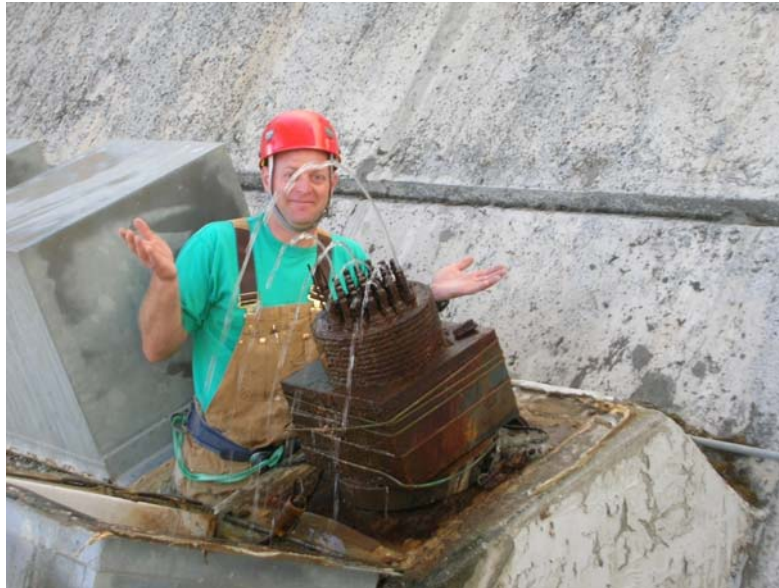
Photograph 1. Water emerging from the free length of an improperly protected tendon subject to excess hydrostatic head (Heslin et al., 2009).
